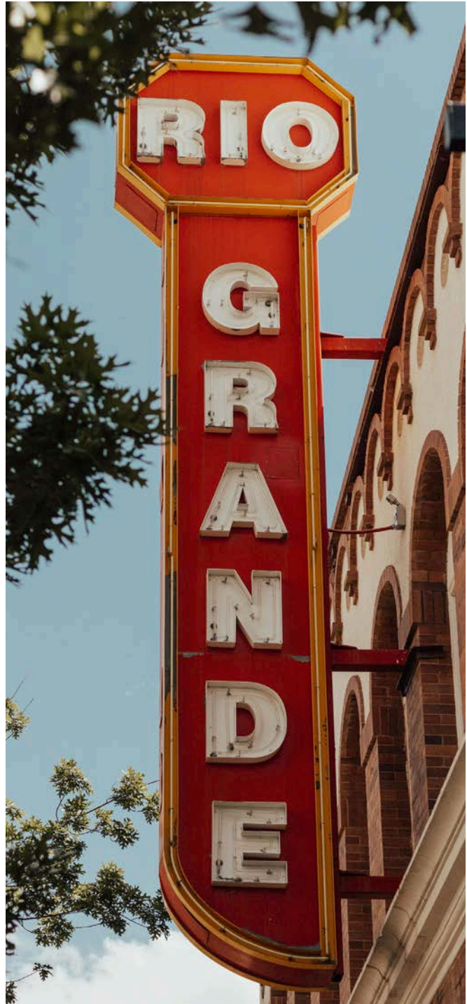
The Rio Grande Theatre (above) in Downtown Las Cruces is listed on the New Mexico State Register of Cultural Properties.
