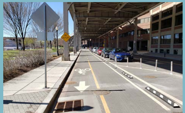
There is no set formula for what a Complete Street looks like, but it should safely accommodate all roadway users.
