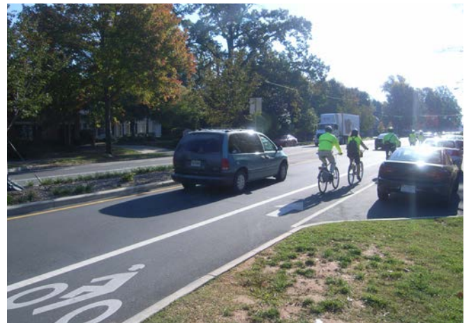
Urban streets can be candidates for lane reductions. The roadway above was converted from a four-lane minor arterial street into a three-lane avenue with on-street parking, bicycle lanes, and intermittent medians (above).
