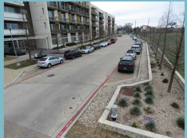
Green streets integrate low-impact stormwater management principles such as permeable pavement and bioretention planters (above).
