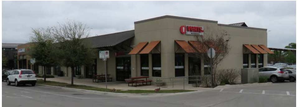
Neighborhood Centers may include single-story and single-use buildings but should be easily accessible to surrounding residents and arranged in a manner that supports and entices pedestrian activity within the roadside.
