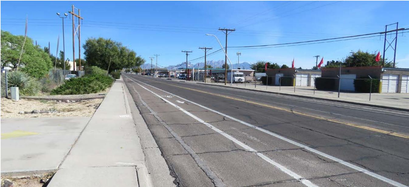
Madrid Avenue adheres to the City's Complete Streets policy by providing sidewalks, on-street parking, and bicycle lanes. The wide street cross-section does little to manage the speed of drivers. The street design and surrounding development patterns do not provide a design context which encourages bicycling, walking, or transit use.
